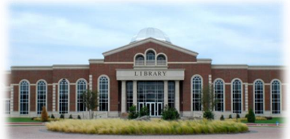
Central Park Campus, McKinney
