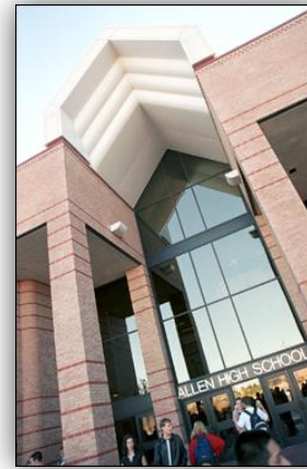
Allen Center 300 Rivercrest Blvd Allen, TX 75002
